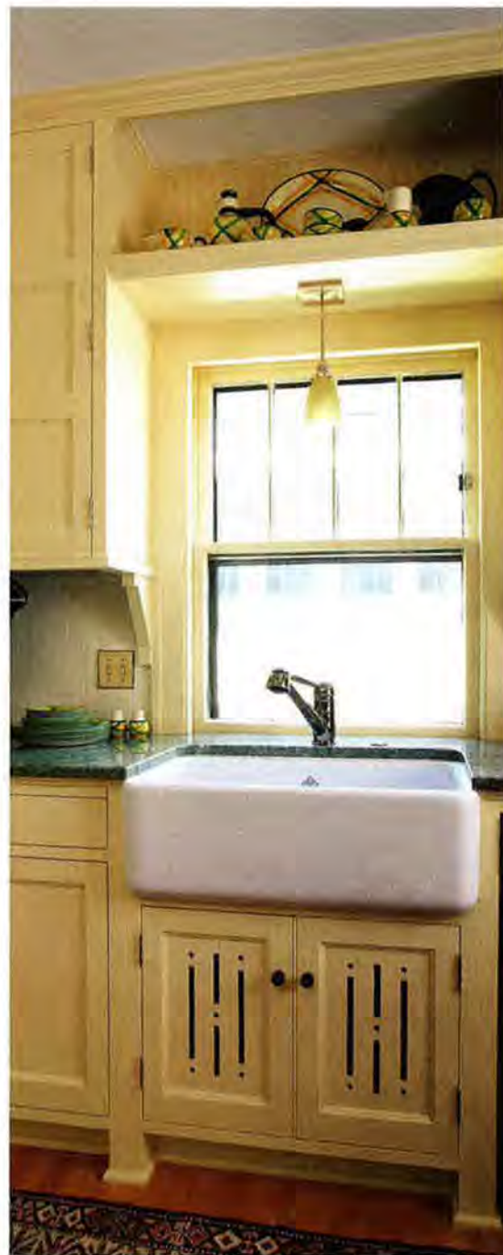
RIGHT: Not all revival kitchens are done in natural-finish hardwoods. This is a new interpretation of the "sanitary" kitchen of the 1920s finished with Benjamin Moore HC-36 Ivory. Note the "Prairie feet" and the vented undersink door with decorative cutouts. David Heide Design Studio renovation.
