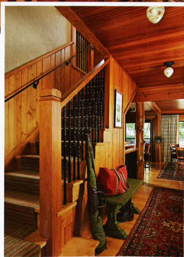
ABOVE Stairs were reversed and rebuilt in a cabin vernacular, with black iron rails made by local blacksmith Clay Beardshear. Lighting was designed and made for the house.
