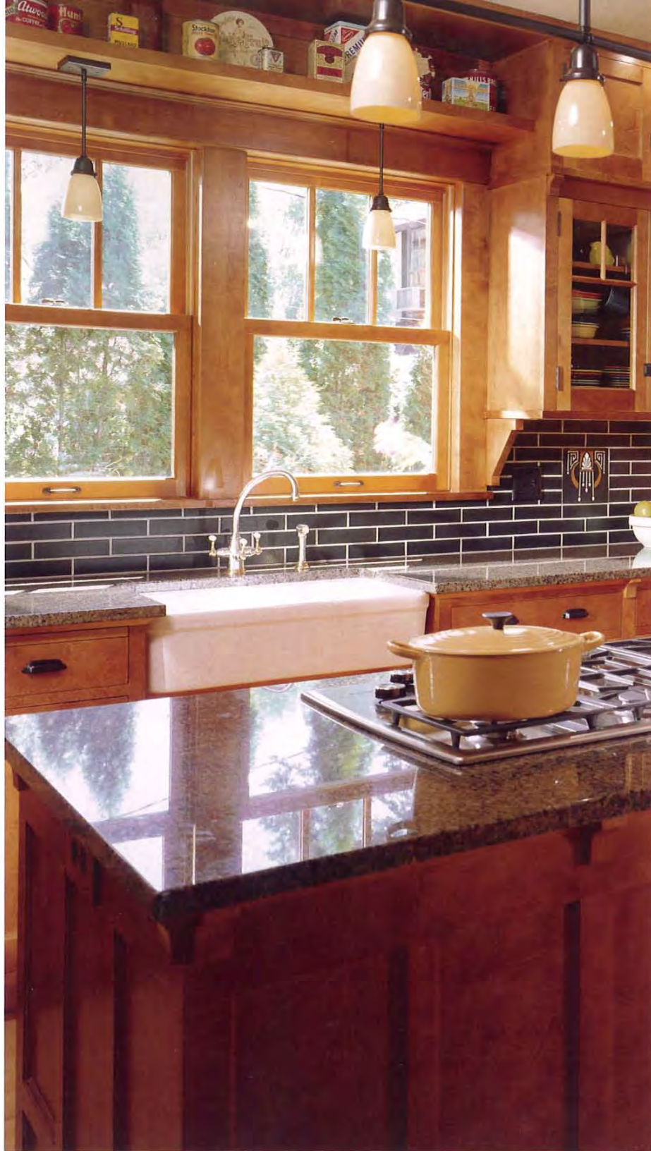
The backsplash wall behind the kitchen sink is composed of historically accurate 2-inch by 6-inch subway tile with custom Arts and Crafts inserts designed and created by Minneapolis-based North Prairie Tileworks.
