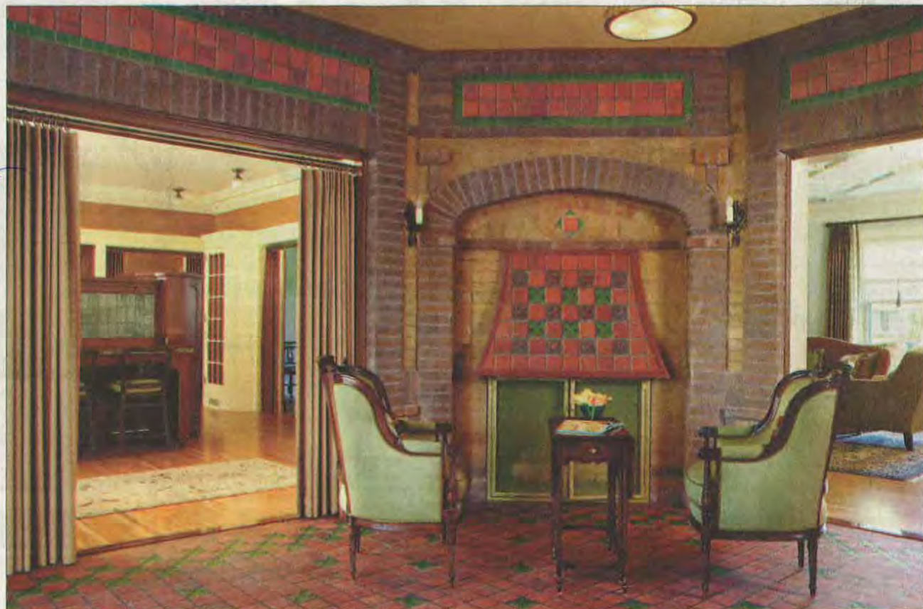
The original brick hood over this fireplace was a clue that there was more decorative detail hidden in the home. The Heide design team replicated the elaborate Arts and Crafts-style brick and tilework, which they discovered buried under drywall, on newly-built walls.
