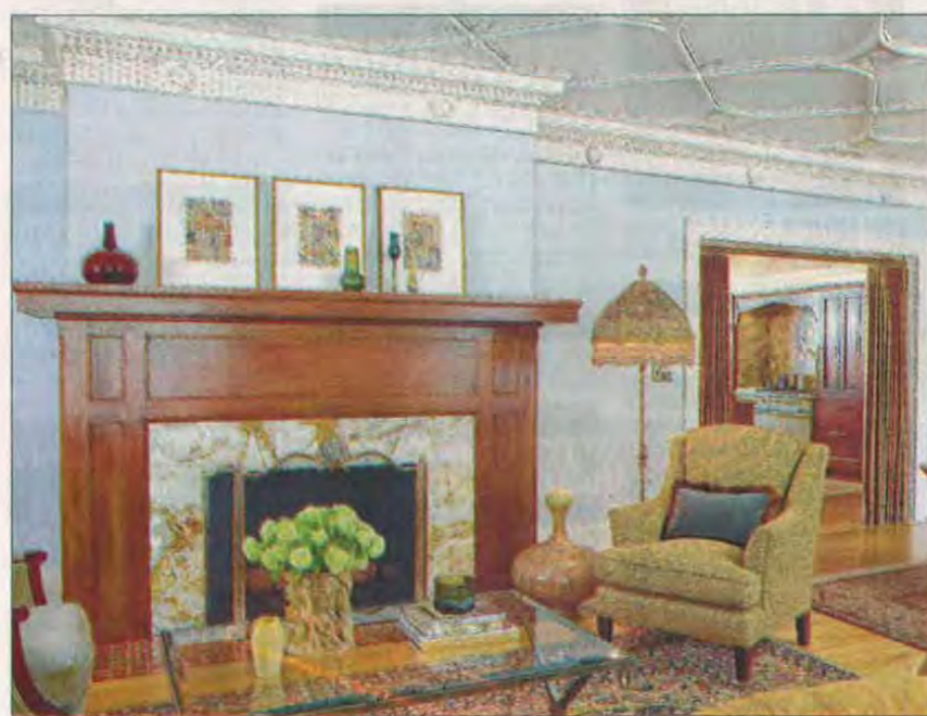
They restored the mahogany mantel, added an onyx surround and rebuilt the decorative plaster ceiling.
