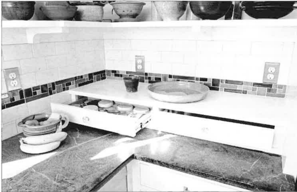
Custom cabinetry creates a space for spices and small items while providing a platform for small appliances. Also, counter space by the refrigerator is preserved. Photo by Greg Page Photography.
