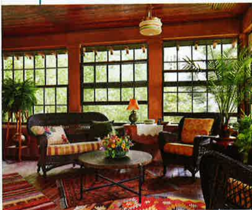
TOP New triple-hung windows follow original proportions. LEFT Several porches on a 1905 lake house had been glazed with high-quality double-hungs that maintain scale.
