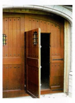
LEFT Cambek built this custom carriage-house door with Tudor styling, even including a wicket, or personsize walk-through door, that allows discreet entry. Closed, the wicket becomes part of the overhead operation.
